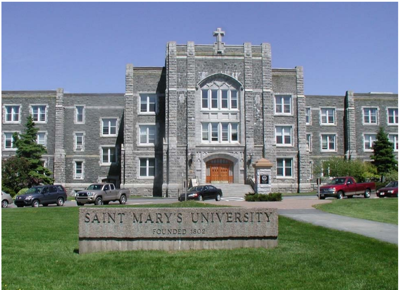
McNally Building, Saint Mary's University
